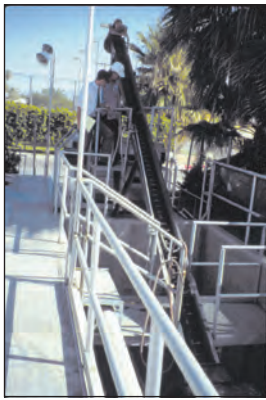
Martin Screw Conveyors are used to remove grit which can be harmful to equipment .
