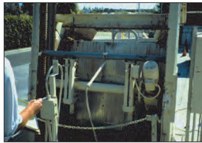
Martin Roller Chain & Engineering Class Sprockets are used in bar screens which removes large debris for transport to the landfill or incineration.
